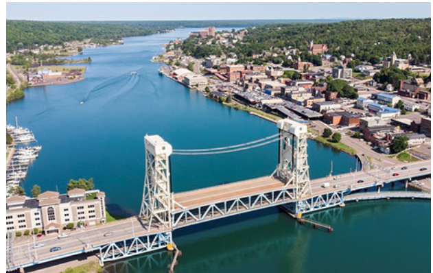
Figure 1. Double-deck Vertical Lift Bridge Example – Portage Lake Bridge, Houghton, MI
