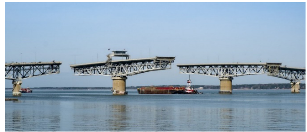
Figure 3. Single-deck Double-swing Bridge Example – Coleman Bridge, York County, VA
