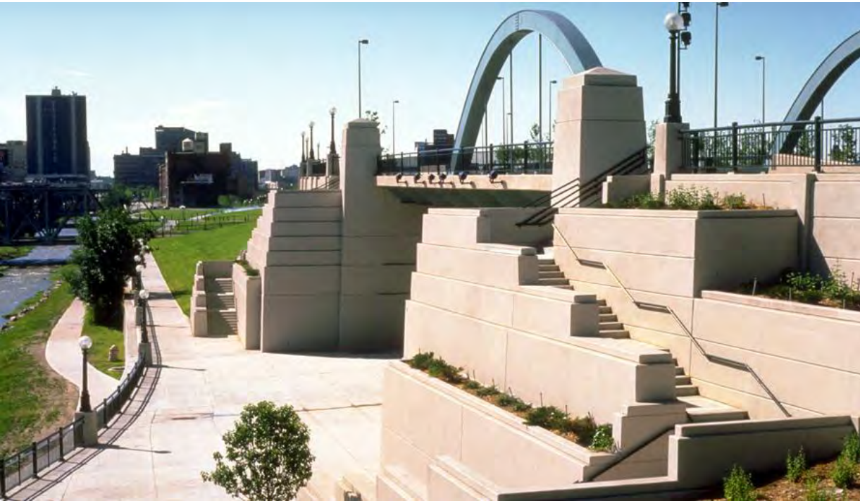
Terraced abutment wall Speer Blvd. Denver, CO
