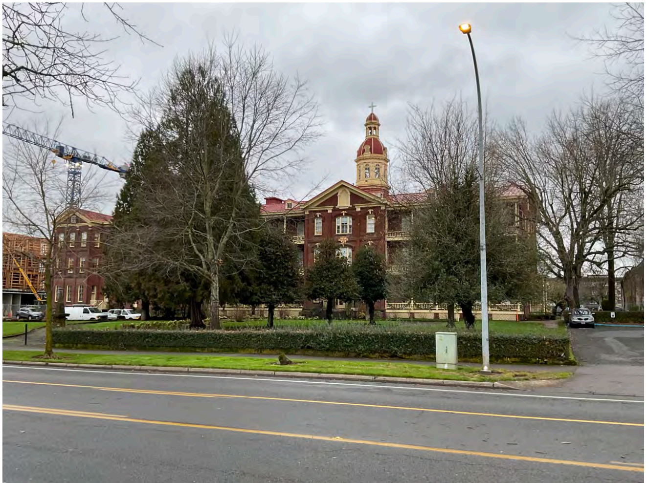
Figure 1. View of House of Providence from south (WillametteCRA 2021).
