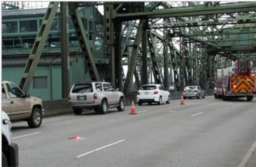
26 Figure 1-2. Crash Blocking the Interstate Bridge
