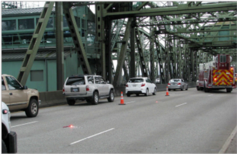
26 Figure 1-2. Crash Blocking the Interstate Bridge
