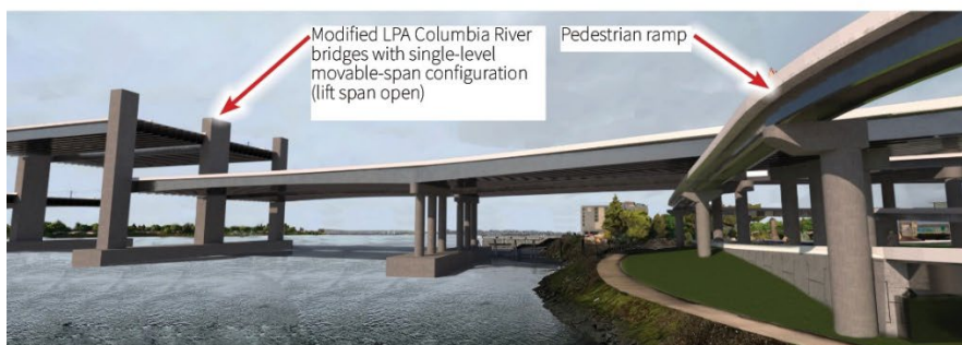
Photographic simulation of Modified LPA with single-level movable-span open configuration with C Street ramp
