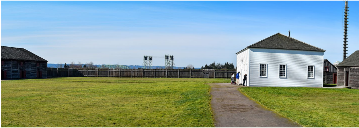
Figure 3-28. Fort Vancouver: Looking Southwest from Inside the Stockade toward the Existing Interstate Bridge (KVP 24)
