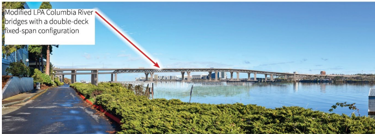
Photographic simulation of Modified LPA Columbia River bridges with a double-deck fixed-span configuration
