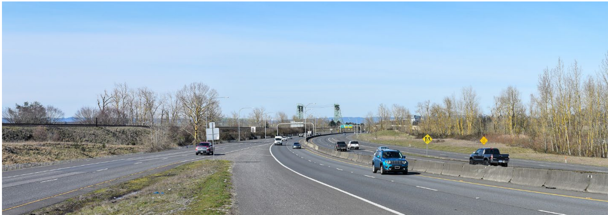
Figure 3-31. SR 14 Westbound: West at I-5 Looking toward the Existing Interstate Bridge Lift Towers (KVP 21)
