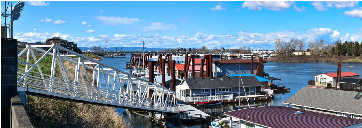
Figure 3-4. North Portland Harbor: West toward the Existing Interstate Bridge (KVP 3)
