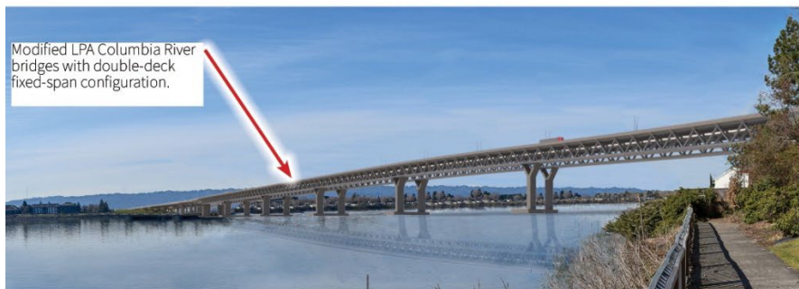
Photographic simulation of Modified LPA Columbia River bridges with a double-deck fixed-span configuration
