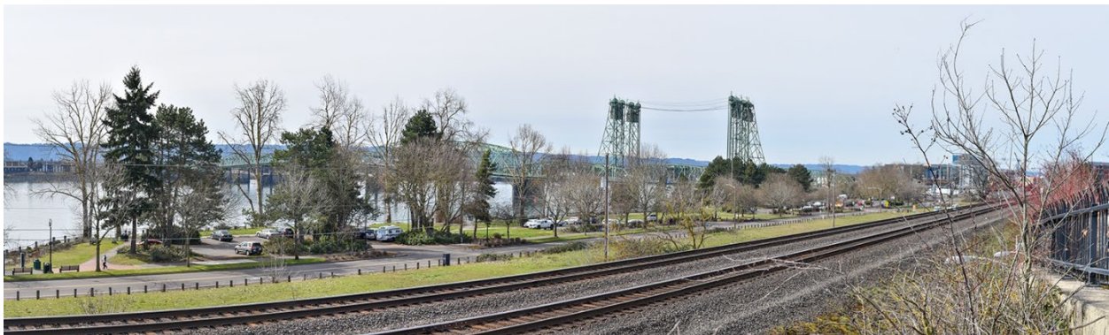
Figure 3-29. Vancouver Land Bridge: Looking Southwest toward the Existing Interstate Bridge (KVP 22)
