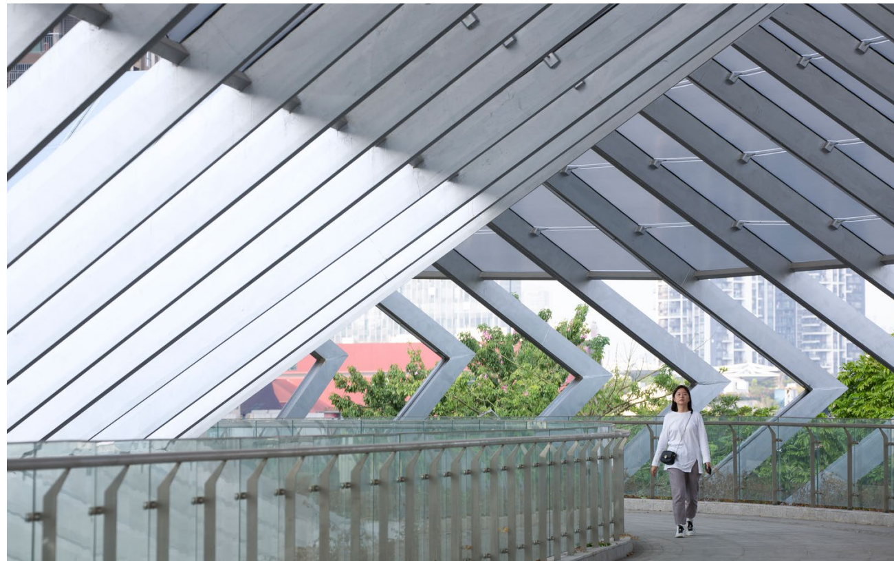
Instead of a utilitarian solution, this raised pedestrian connection feels inviting, safe, and welcoming.
