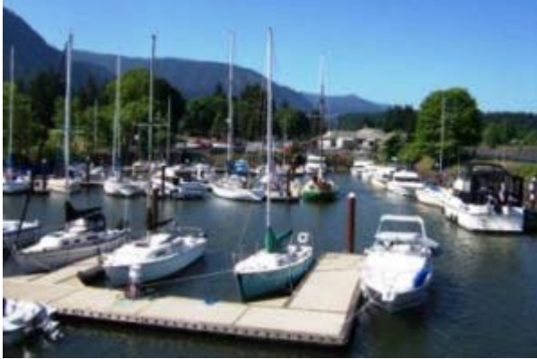
Figure C.2-26. Port of Cascade Locks Marina
