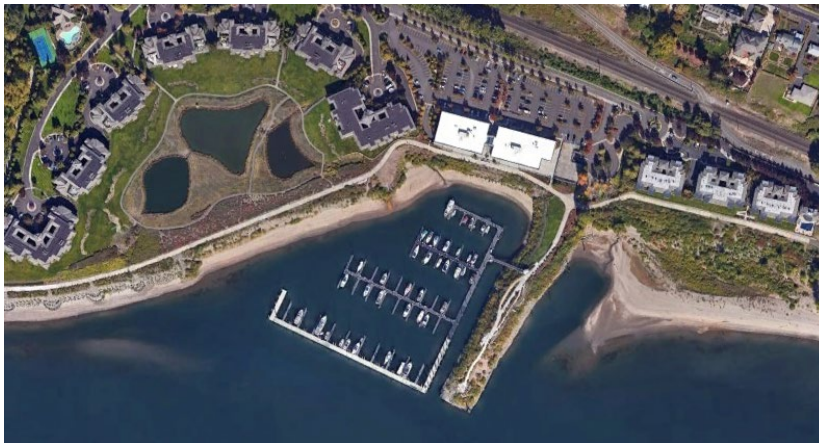
Figure C.2-3. Tidewater Cove Marina
