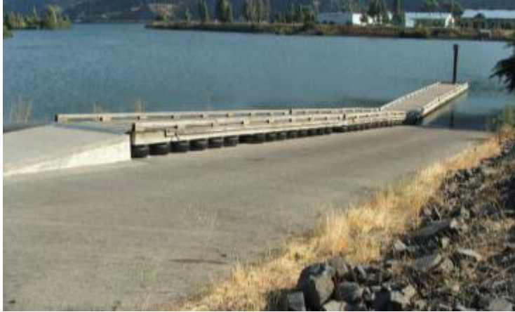
Figure C.2-17. Port of Klickitat Bingen Marina
