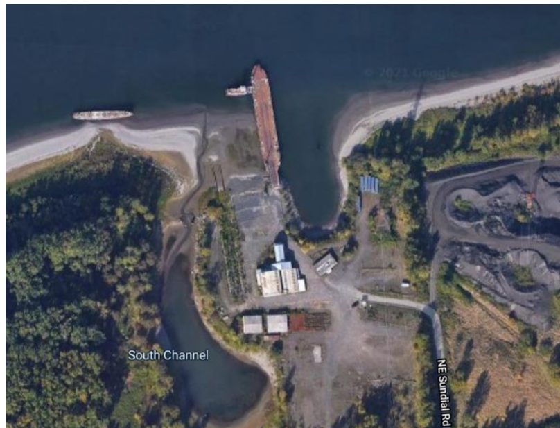
Figure C.2-22. Sundial Marine Tug & Barge Works
