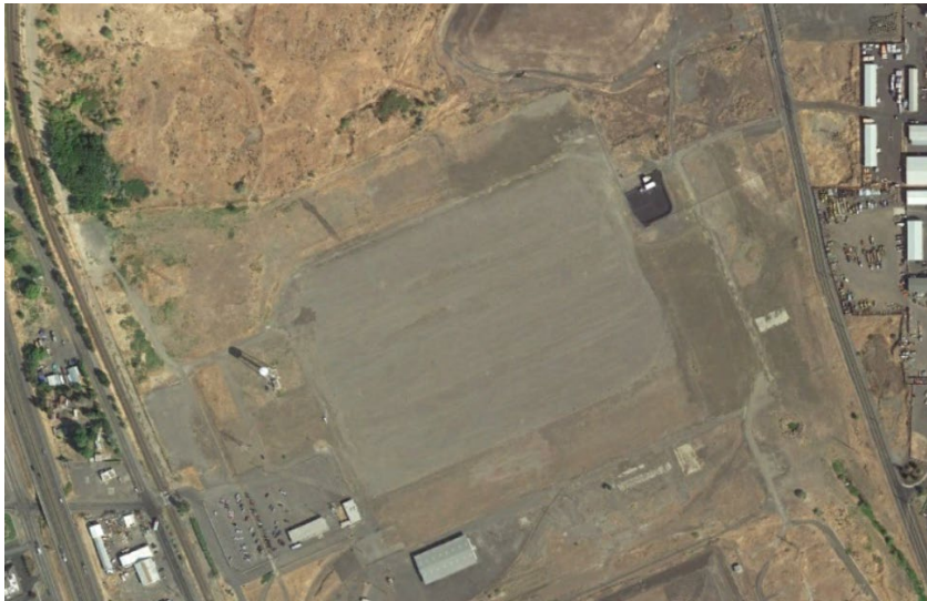
Figure C.2-33. Former Northwest Aluminum Site (3313 West 2nd Street)
