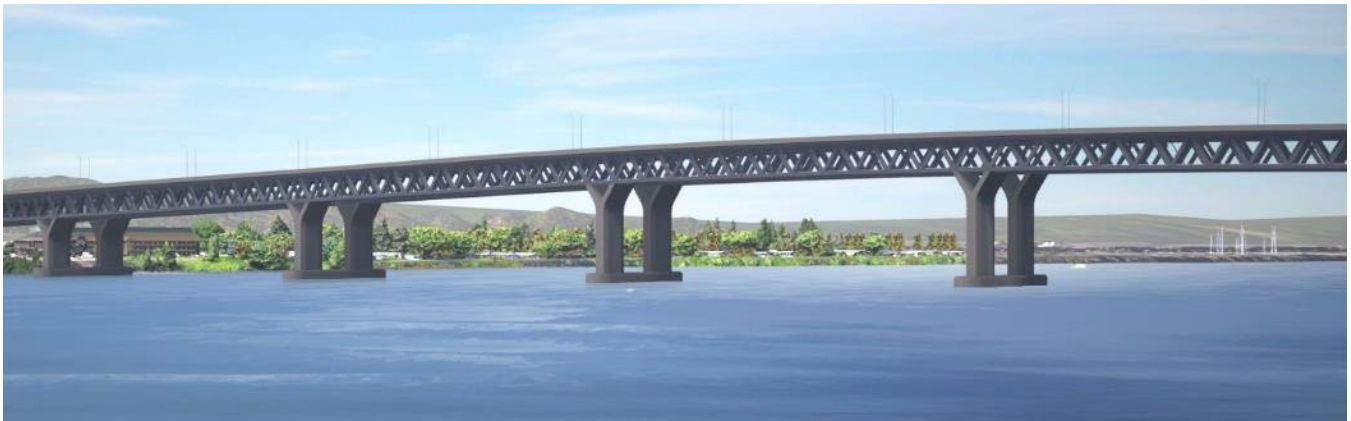
Figure 3-11. Example of a Double-Deck Fixed-Span Truss Bridge
