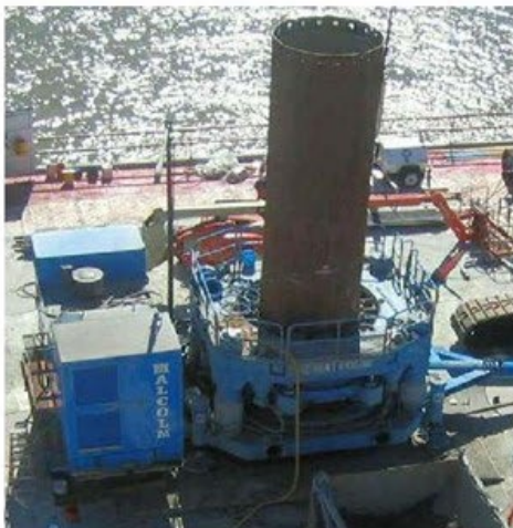
Typical Water-Based Drilled Shaft Installation
