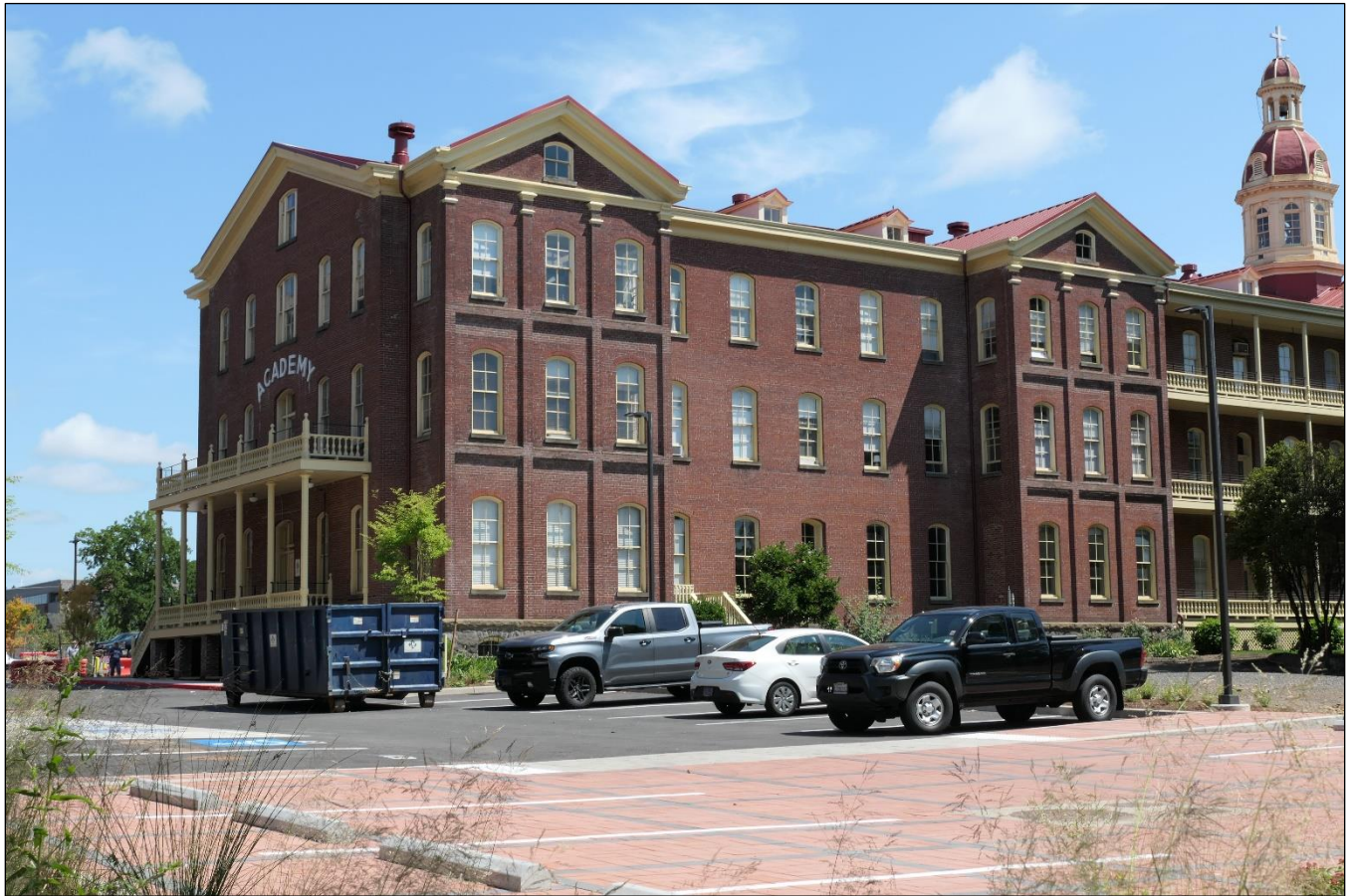
Figure 4. View of House of Providence 1891 addition from southwest (WillametteCRA 2023).
