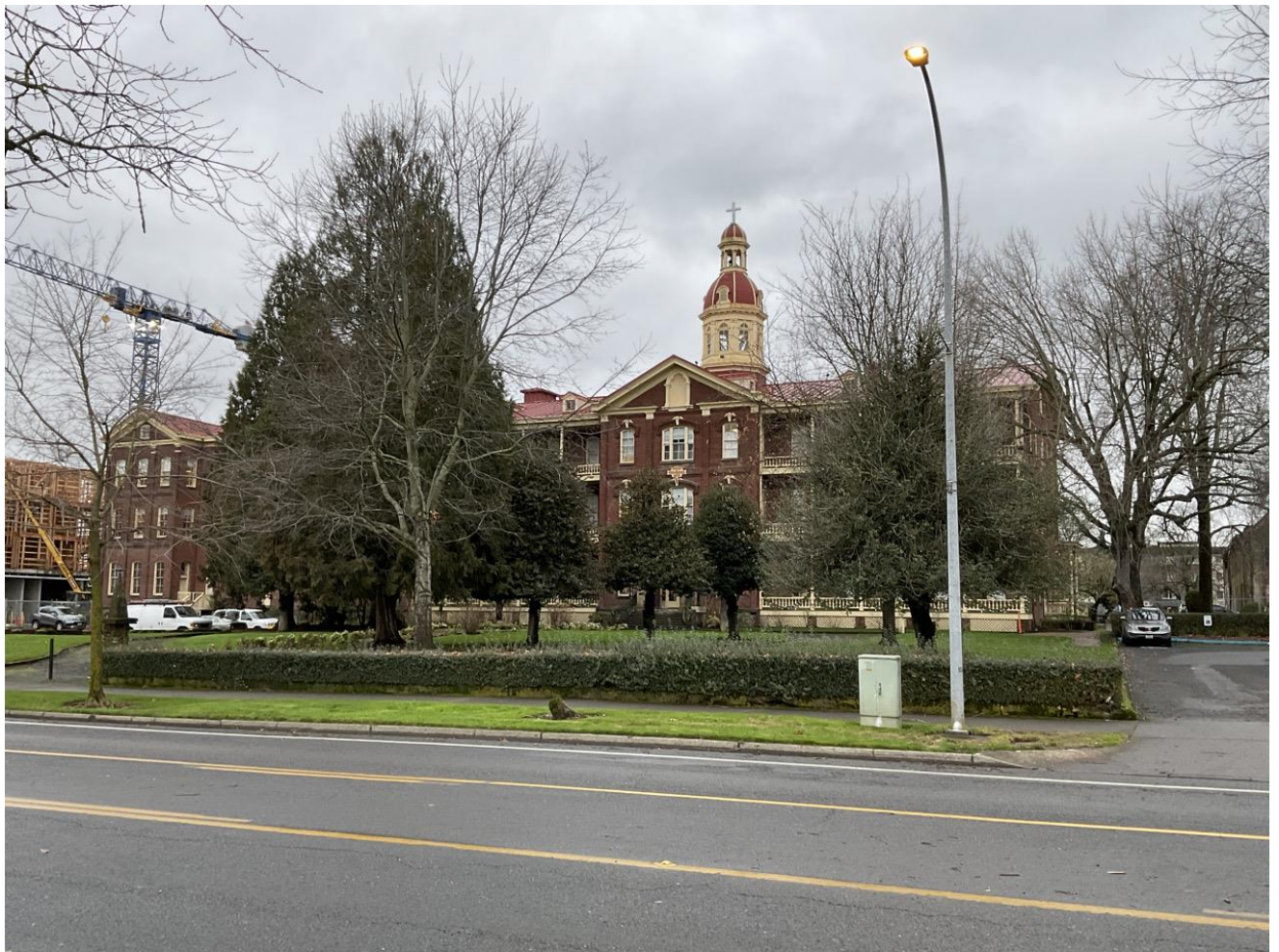
Figure 1. House of Providence, view from south (WillametteCRA 2021).
