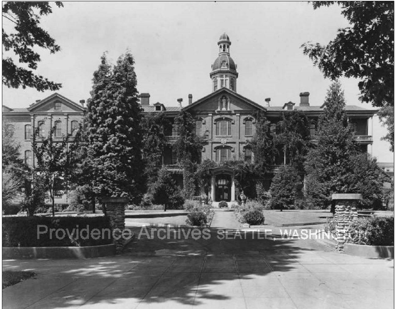
Figure 13. View of House of Providence ca. 1920s from south (Providence Archives, Seattle, Digital Collections).
