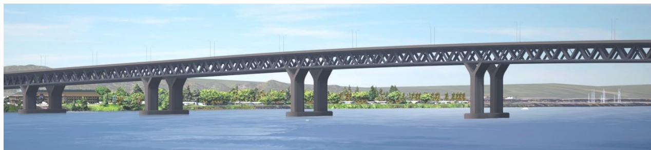
Figure 1-15. Conceptual Drawing of a Double-Deck Fixed-Span Configuration
