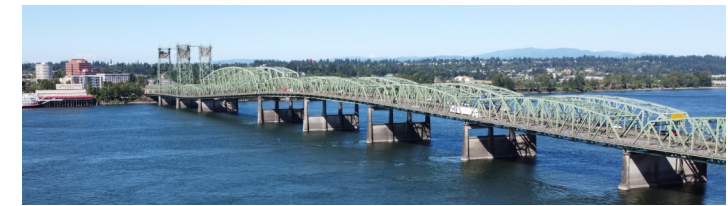
104-year old I-5 Bridge
